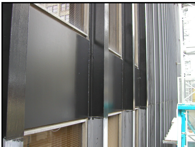
Freshly painted exterior surface
